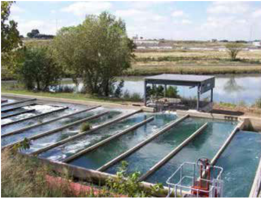
Figure 6.6: Chlorination Basin & Schematic Diagram of Chlorine Dosing & Mixer
