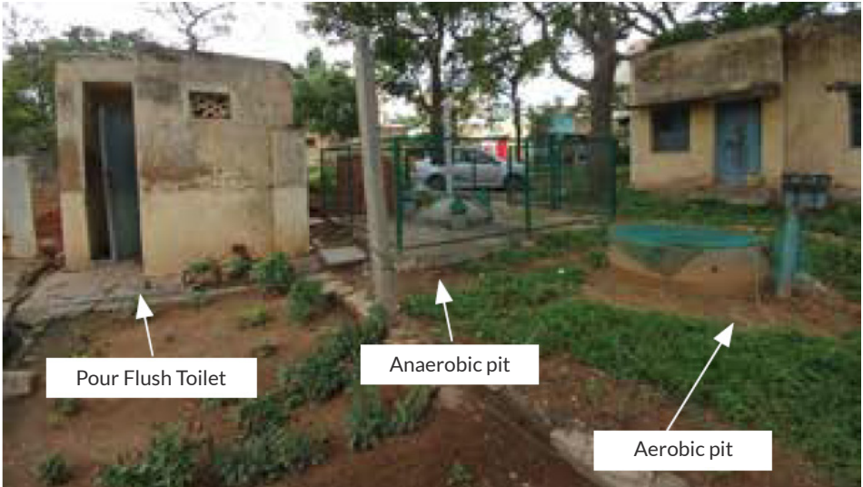
Figure 5.5: A PRB Twin pit toilet at Mulbagbal Town, Karnataka
