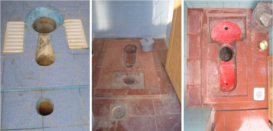
Figure 4.4: Ecosan toilets in Bangalore, Dhanduka (Ahmedabad) and Rayka (Vadodara)
