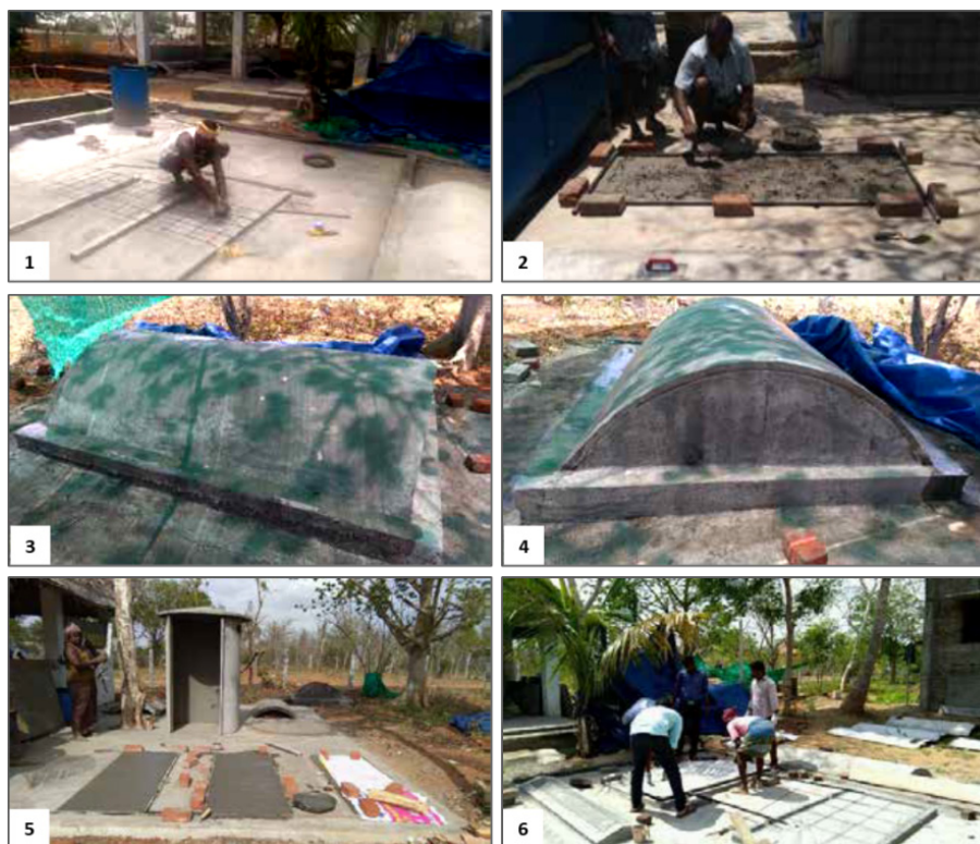
Figure 4.13: Step by Step Installation Process of Sunidhi Toilet
