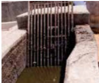
Figure 8.8: Bar screen at Niayes faecal sludge treatment plant, Dakar, Senegal
