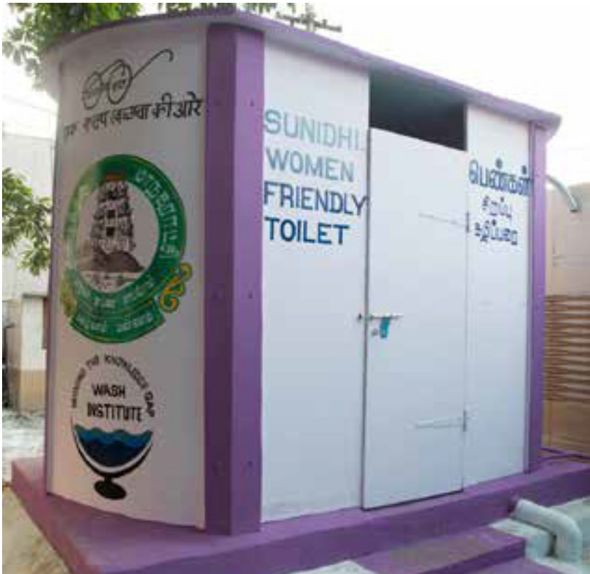
Figure 4.12: Sunidhi Toilet installed in public space
