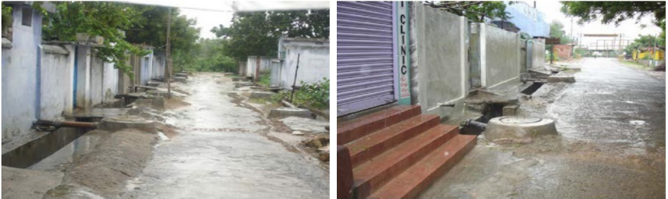
Figure 5.27: Simplified sewer with shallow chambers in a housing colony
