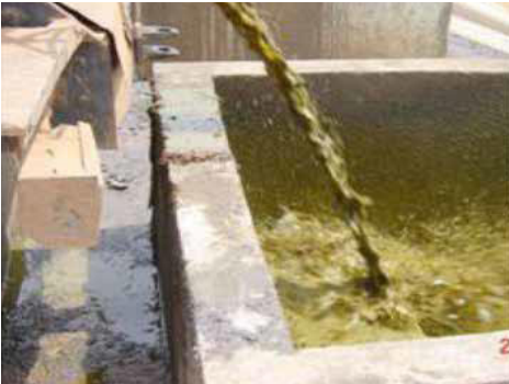
Figure 8.6: Faecal Sludge being emptied at a FSTP
