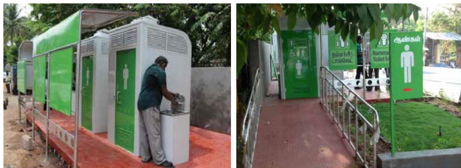
Figure 4.11: Views of Installations in public spaces
